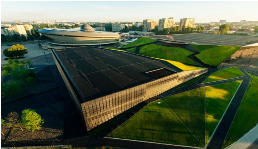
Internacional Congress Centre in Katowice
